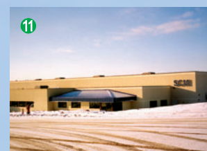
Sumitomo Electric Carbide Manufacturing, Inc. (Established in 1991 / Milwaukee, U.S.A.) Production of Multidrill, CBN and PCD cutting tools.
