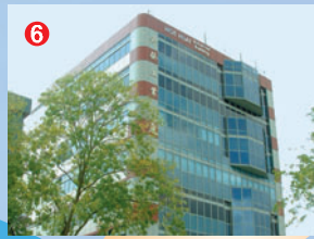
Sumitomo Electric Hardmetal Asia Pacific Pte. Ltd. (Established in 1998 / Singapore) Sales and marketing headquarters for South East Asia market.
